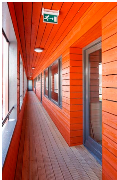
→ Access to the walkway at the rear
